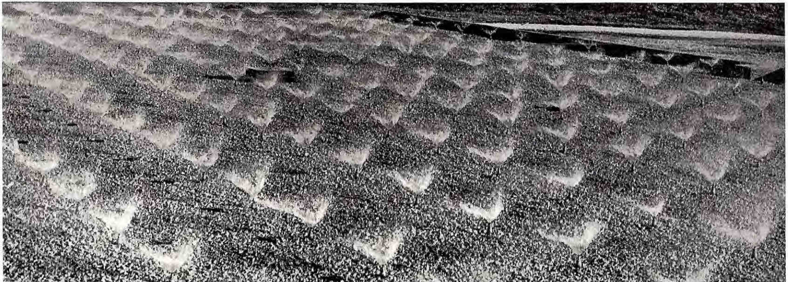
Sprinkler heads distribute partially treated sewage over a bed of limestone, at the Miller treatment plant, where a biological action by aerobic bacteria takes place.
