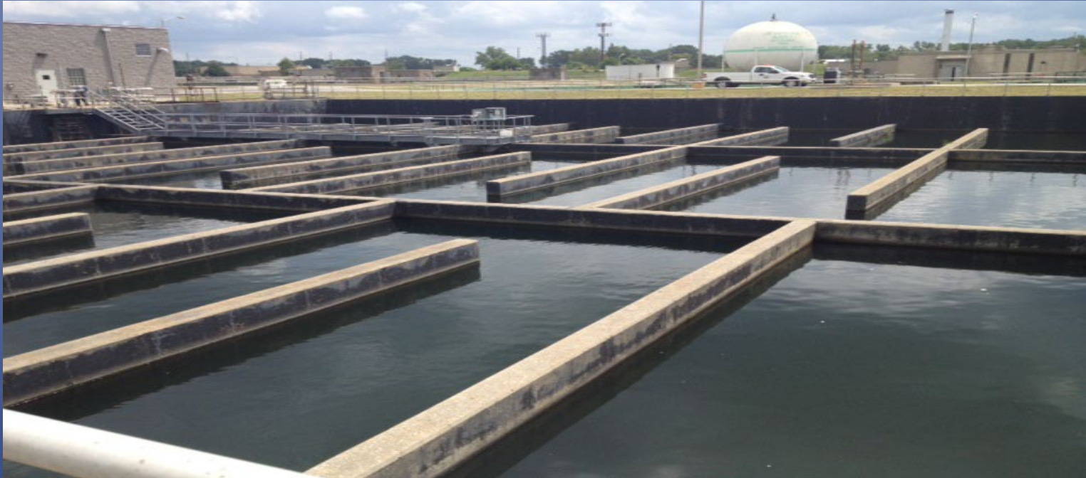
Chlorine Contact Chamber
